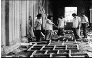
Fig.3. Restoration work in Raja Rammohun Roy's house
